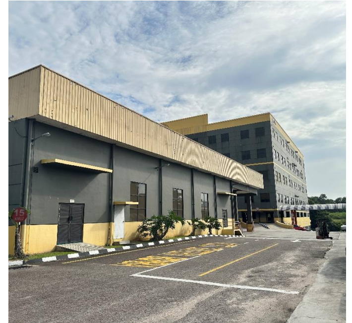
SRX factory in Johor Bahru, Malaysia.
